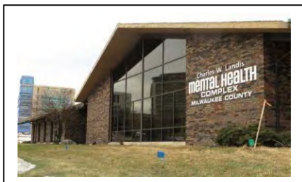
Milwaukee County Mental Health Complex
