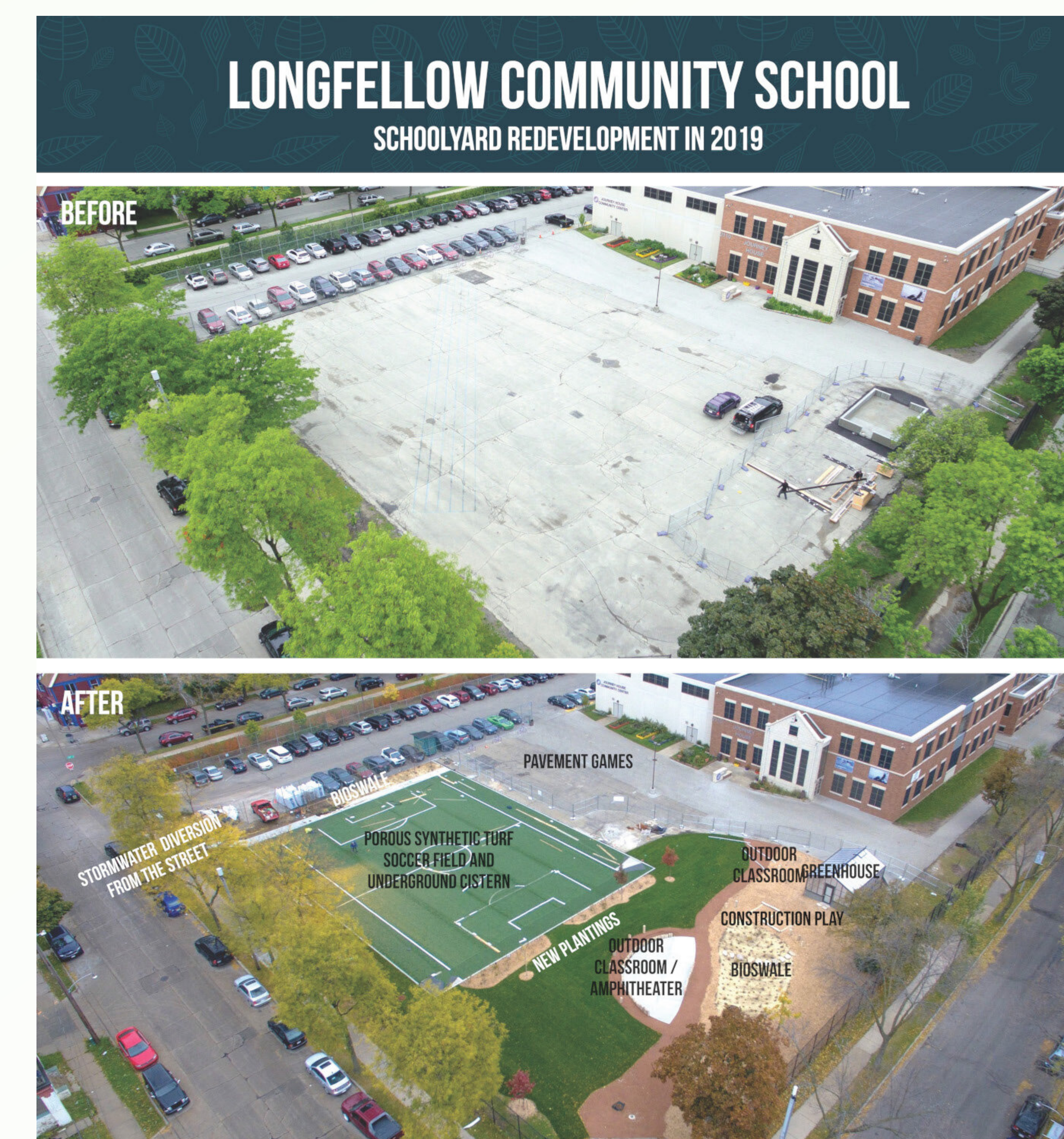
Figure 2. Photos of Longfellow School schoolyard before and after construction of green schoolyard
