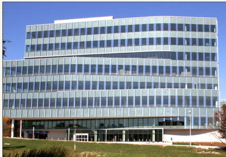
The Center for Advanced Care, the newest addition to the Froedtert Hospital campus.
